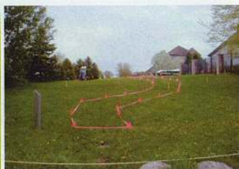
The buffer planting beds and path are laid out.
